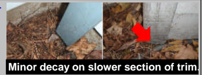
Decay at front entry trim board.
