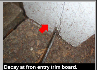
Decay at front entry trim board.
